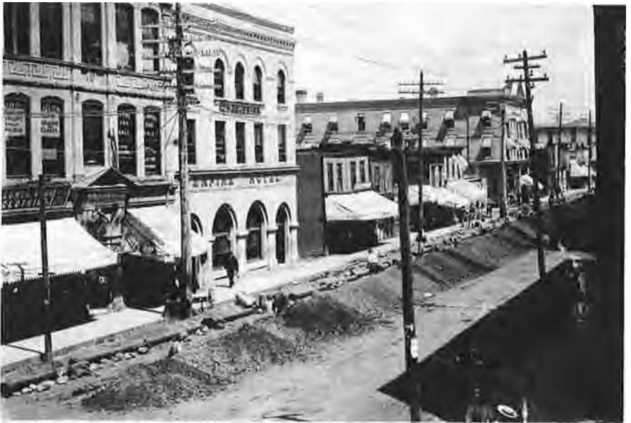
Constructing a sewer line on Rosser Avenue
