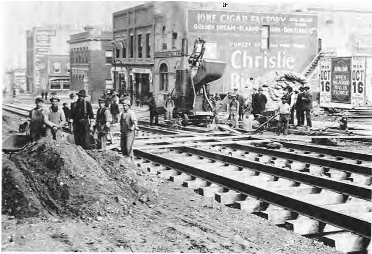
Street railway construction, Oct. 1911.
