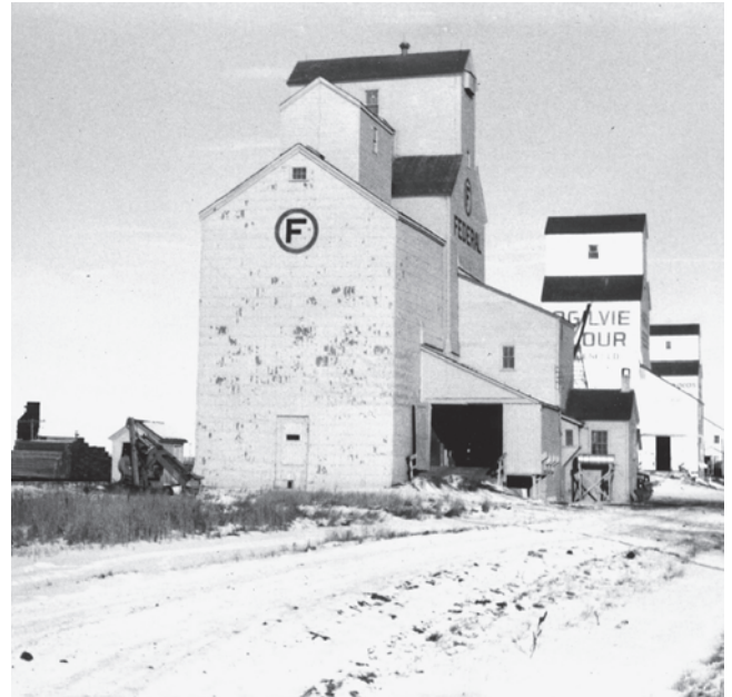
Rosenfeld's grain elevators in the late 1950s. [George Fast] The narrow black structure in the distance on the left is the coal dock, used by CPR steam engines to fill up with coal.
