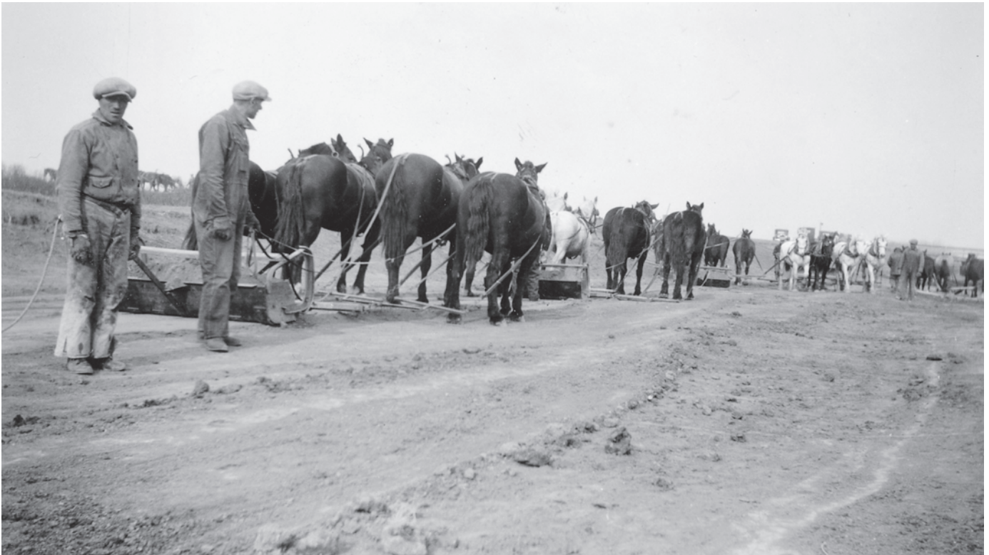
Road gang working on Highway #14A, now #30, near Rosenfeld. Undated. These men are using Fresno scrapers with teams of four horses to smooth the road. The Fresno scraper was invented in 1883 by James Porteous in Fresno, California. It would scoop up the dirt and was controlled with a lever to cut deeper and also to dump the dirt. Note: Paving of these highways started in the mid-1950s. [Judy Fehr]
