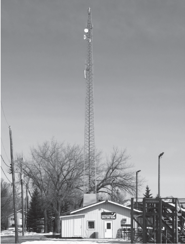
In the fall of 2014, Valley Internet Provider (VISP), the first fibre-optics-based wireless Internet provider in the area, erected its tower in the town of Rosenfeld. [Art Wiebe]
