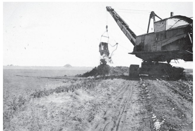
Digging the double dyke near Amsterdam S.D. [Paul Reimer]
