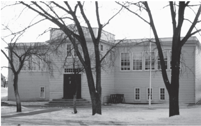
The 1937 "Coronation School" on Acheson St. in Rosenfeld (1970). [Arnold Mekelburg]
