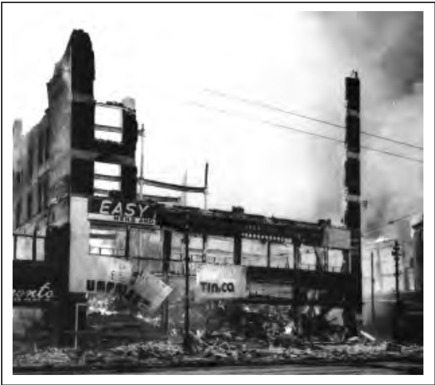
The day after the Time Building fire of June 8, 1954.
