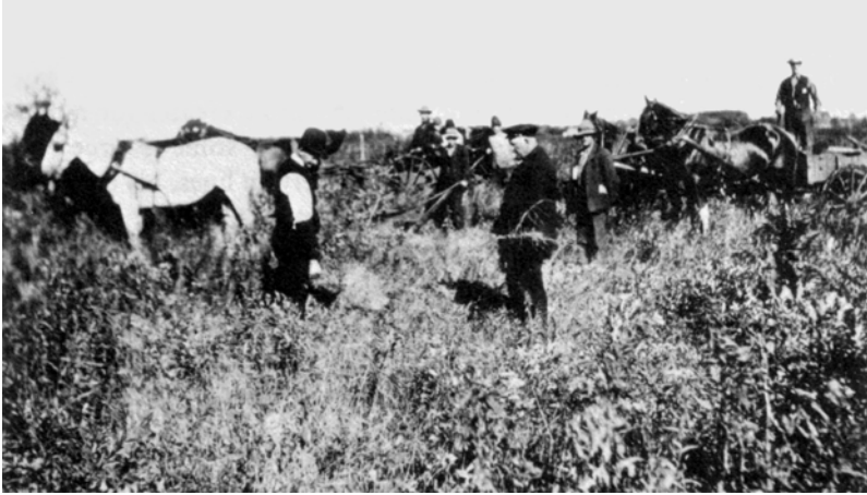
Cotton and the Reverend W. J. Lobb turning the first sod for the Methodist Church at Kenville, 1912.
